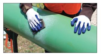
4.4 NOTE: Premier Bore-Wrap is not an anti-corrosion coating, thus the mainline and field joint coating should be inspected for holidays prior to applying Premier Bore-Wrap so that repairs can be made.
