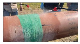
6.3 Premier Bore-Wrap is a water activated wrap. It is necessary that water is continuously sprayed onto the surface and underbelly of the roll as it is being applied. You cannot oversaturate the material, however insufficient water will slow the reaction and reduce product performance.
