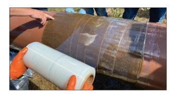
6.7 Once fully compressed, use the perforating tool to puncture the compression film. This will allow for excess resin, moisture, and  $CO_2$  from the reaction to escape. Perforate using enough pressure to get through the compression film but not through the layers of Premier Bore-Wrap.
