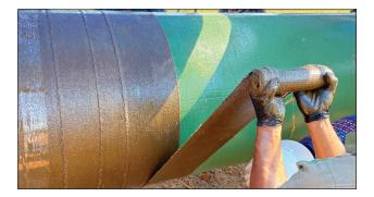
6.6 Ensure the wrap is completely saturated and then immediately begin wrapping compression film over the Premier Bore-Wrap quickly and with tension applied. Overlap each end of the Premier Bore-Wrap by at least 6" (150 mm) to ensure the ends lay flat and the resin can be retained. 3 passes will provide sufficient compression.
