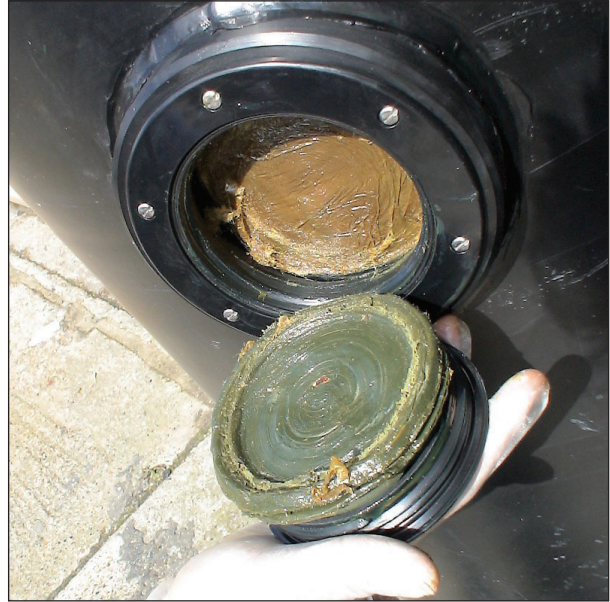
A threaded cover is removed to expose the Petrolatum tape layer used in the SeaShield 2000HD or 2000FD System. The internal area of the port is filled with a petrolatum filler to exclude water and other marine growth.
