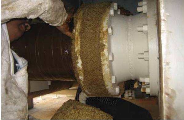
Prembond Mastic will adhere to metal, PVC, polyethylene and concrete.
