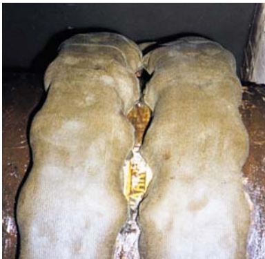
Premier Molding Compound Blankets applied to flange pair.
