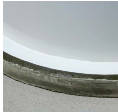
Premier Molding Compound applied to protect tank bases from corrosion.
