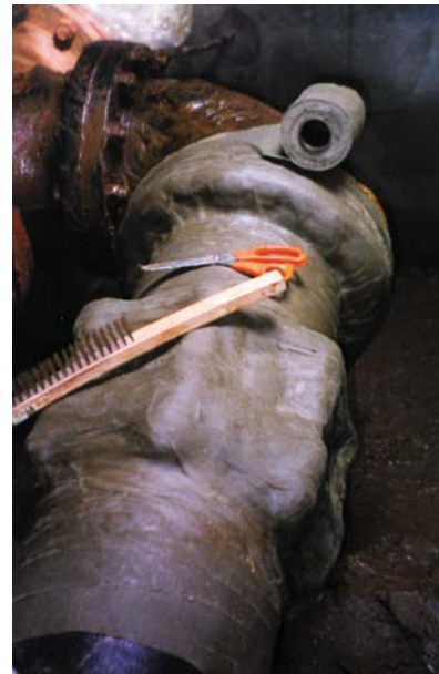
Complete corrosion protection of pipe, flange and coupling.
