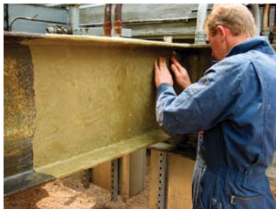
Petrolatum Tape system (Prembond Hi-Tack Tape) applied to structural steel.
