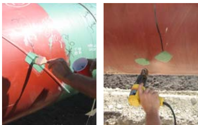
Protal Repair Cartridge application.
