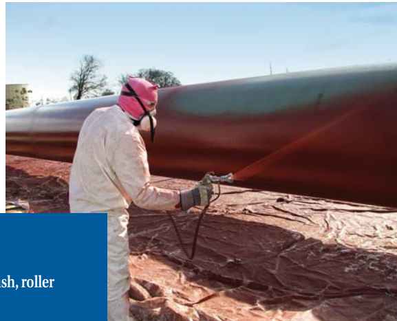
Protal ARO being sprayed applied.
