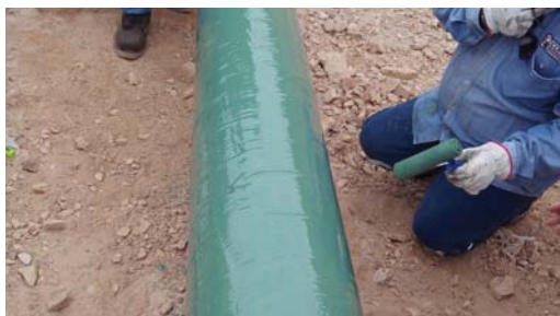
Protal 7200 applied to section of pipe in rocky soil.
