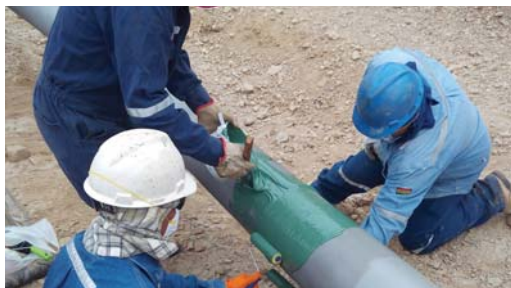
Application of Protal 7200 using a roller.
