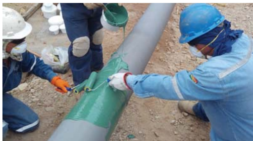
Application of Protal 7200 in one coat at 50 mils.
