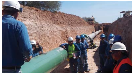
Protal 7200 already applied in part of the pipeline.
