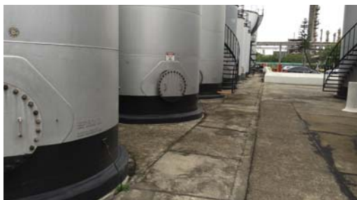
Several tank bases fully protected from corrosion.
