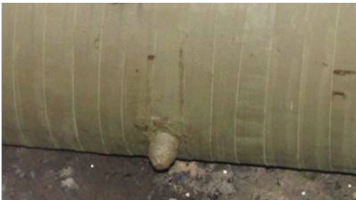
Premtape Tropical already applied on difficult shapes on the pipe.
