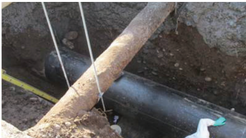
Contractor applying Prempaste to pipe substrate.
